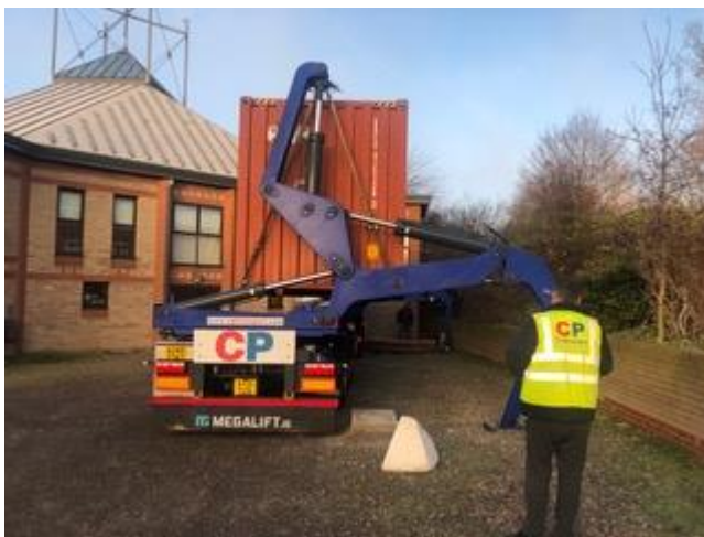
The container being unloaded on site
