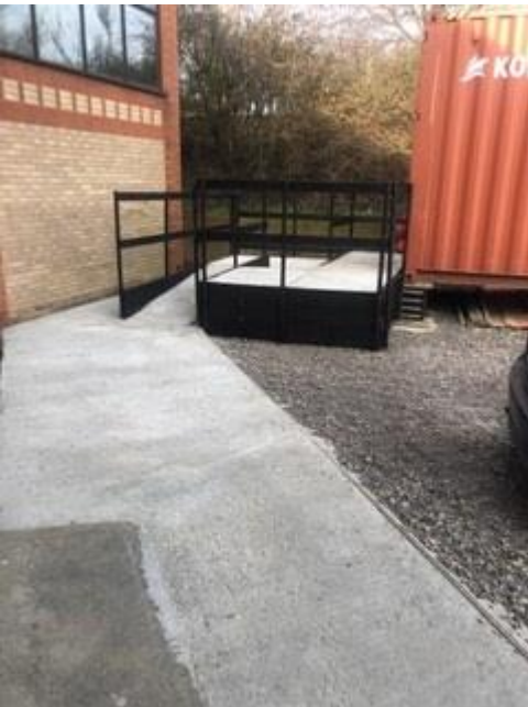
Concrete and ramp finished
