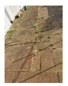
Prior to repairs. Broken and uneven paving causing trip hazards
