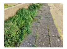
Most of the walkways have been overhauled on a piecemeal manner over the past 12 yrs as our own funds have allowed. During season 2022/23 it was noticeable that the St Edmunds side walkway had deteriorated to a point where trip hazards had been created due to movement and cracking of the paving therefore it became a critical and priority activity to rectify the problem.
