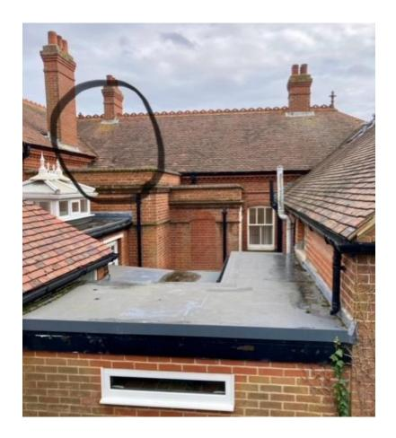
There is a slipped/broken tile just below the far right side, apex chimney, a trick area to access. However, as the rosemary/plain tiles provide such coverage that it prevents meaningful water ingress, it is suggested that this is left alone.
