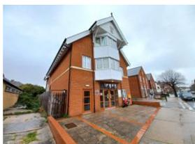
A detached three-storey building within a conservation area providing space for day centre on the ground floor, with residential flats above. Pitched roof covered in slate with dormer windows, facing brickwork with timber cladding.
