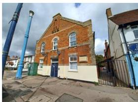
A detached two-storey building originally built in 1886 with a modern extension completed in 2007. Community hall on ground floor with residential flats above. Pitched roof covered in slate, dormer windows, Velux roof lights. facing brickwork with timber and UPVC windows and timber entrance doors.
