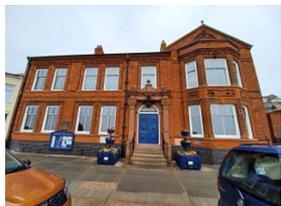
A two-storey building within a conservation area. Pitched tiled roof with chimney stacks, facing brick walls with decorative frieze and entrance door, timber sash windows.
