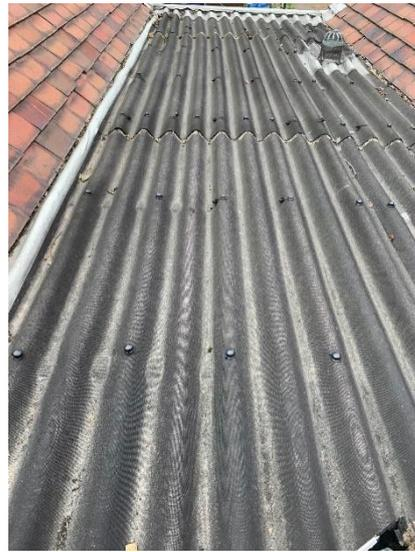
The black roof that covers the area outside the Cemetery Workshop is deteriorating, especially the flash band that has gone very brittle and is in places allowing water through in small amounts. There are also cracks appearing in the bitumen sheets. Again although the staff are not experienced in this they are willing to tackle the job, however, it would likely take a week's work and the cost of materials to purchase would come to approximately £600.
