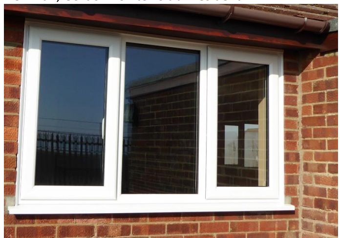
One of the replaced windows at the rear of clubhouse
