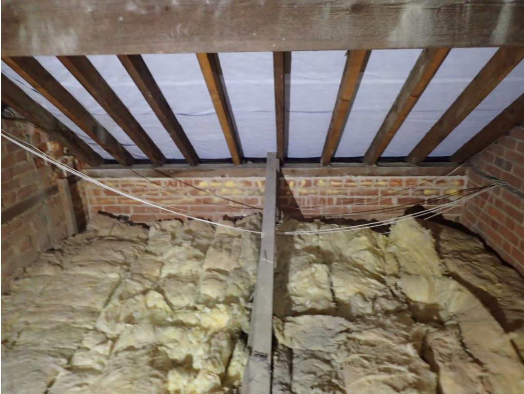
MIDDLE OF FRONT ELEVATION BRICKWORK
