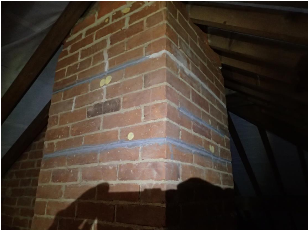
RIGHT (SW) CHIMNEY, HELI BAR TIES BEHIND CONTRASTING MORTAR
