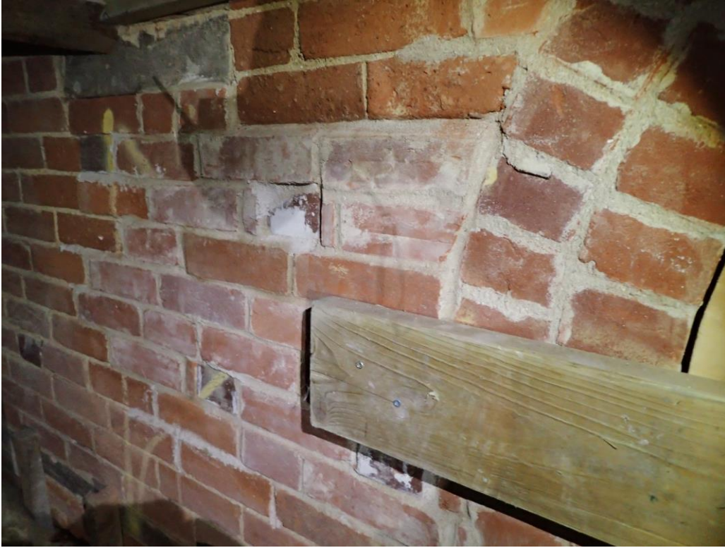
BRICKWORK MADE GOOD EITHERSIDE OF ARCH
