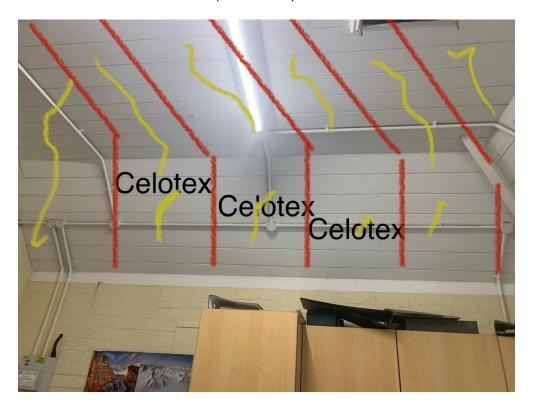
This method of baton and boarding can also be used to address the issue of the high joists in the workshop to ensure the whole roof area is insulated, and also address the issue that in the main Cemetery office the access is very small about 30cm x 30cm so it would restrict getting materials up there.
