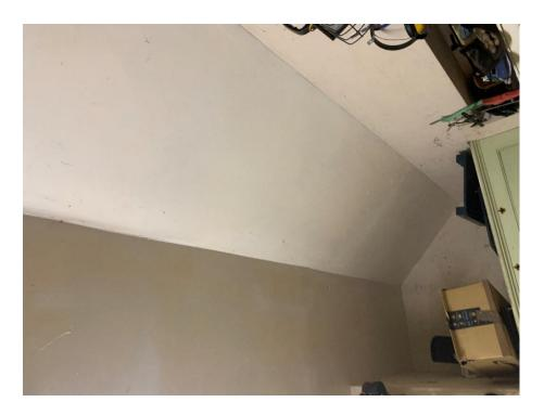
One method to prevent the cold spot would be to put in batons and then insulate between them and reboard (see below)
