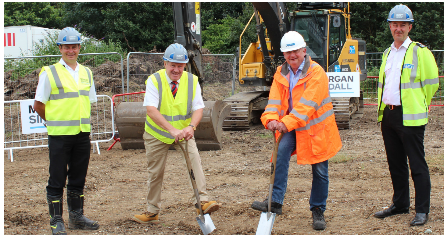
Pictured above: (l-r) Deputy Fire Chief, Dan Fearn; Tim Passmore; County Councillor Andrew Reid and Chief Constable, Steve Jupp officially mark the start of works of Stowmarket Fire Station in July 2021.
